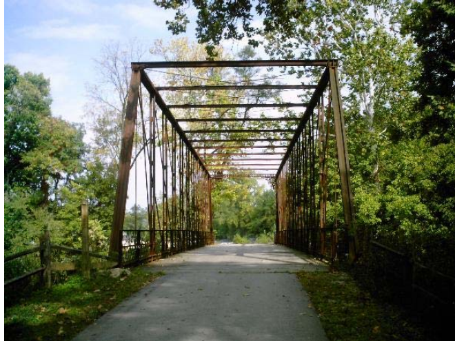
Old U.S. 36 bridge crossing White Lick Creek
